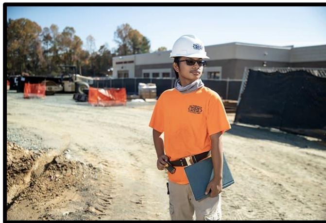
Christopher Borja, youth apprentice with Altimate Electric, Inc., at his worksite Hammond High School, a Howard County Public School System facility.
